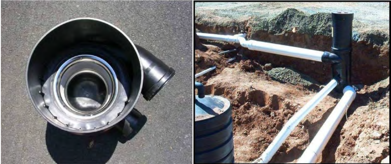
Figure 4.6.9. Interior of Vortex (left) and Installation of Vortex Filter Prior to Backfill (right)
