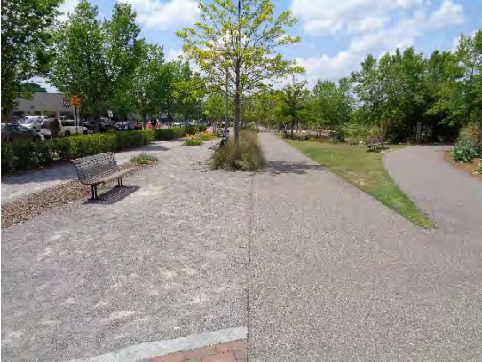
Figure 4.4.1. Permeable Pavement incorporated into sidewalk design
