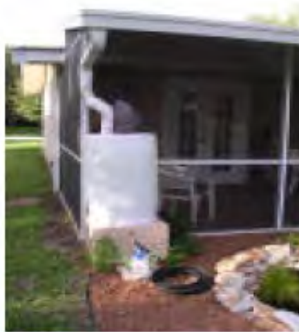
Figure 4.6.3: Type 1: Rainwater Harvesting with a Rain Barrel
