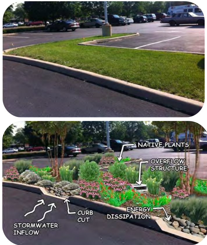
Figure 4.1.2. Bioretention – Before and After Parking Lot Island
