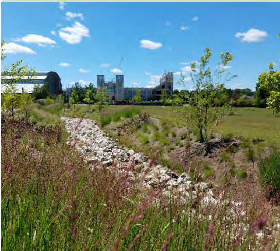
Figure 4.3.1. Example of Dry Water Quality Swale
