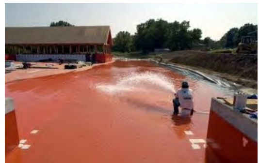
Figure 4.7.4. Flood Testing the Waterproofing Layer
