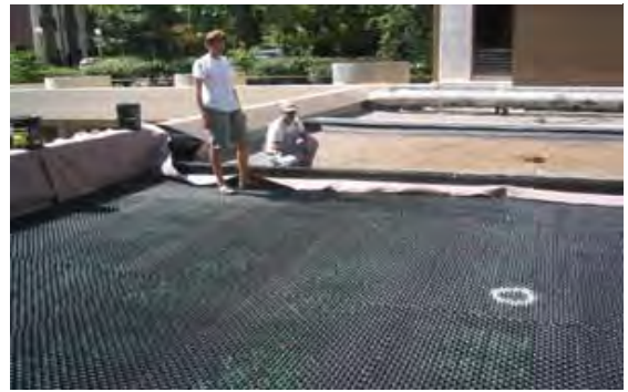
Figure 4.7.5. Drainage Layer Installation
