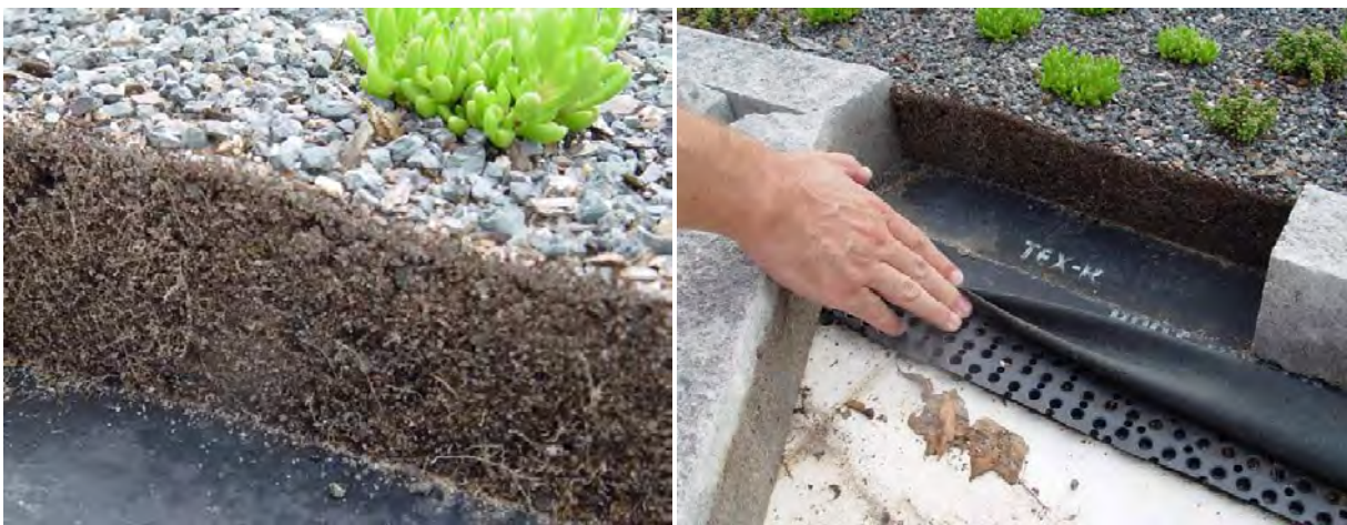
Figure 4.7.3. Greenroof Cross-Sections
